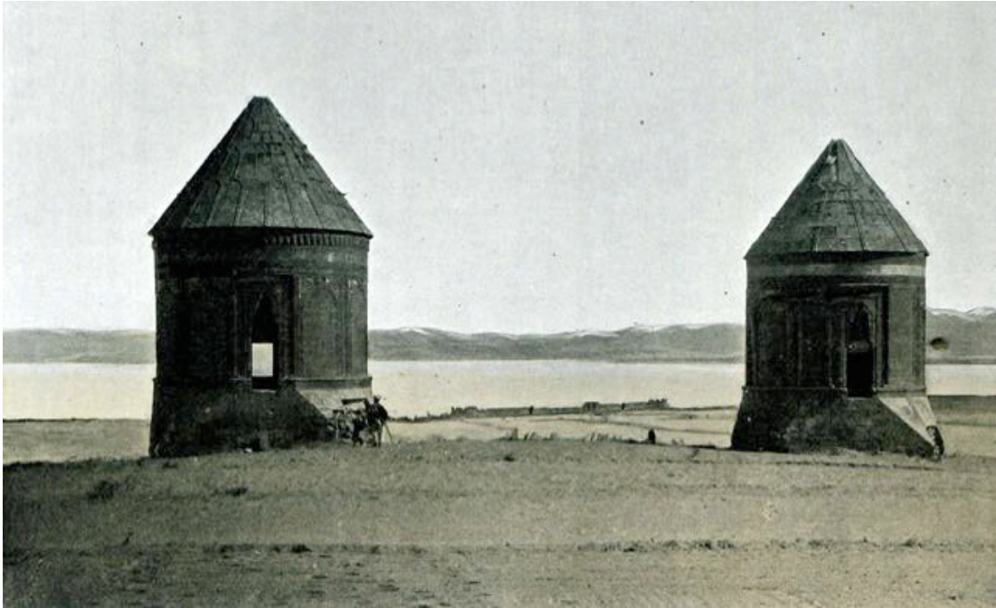
Fig. 11: İki Kubbe tomb towers, view from the north with the Ottoman citadel in the distance (source: Lynch, Armenia , 285)
